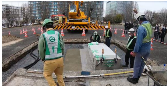
(c) Setting Precast Coil
