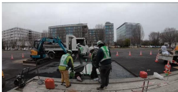
(e) Paving with Asphalt
