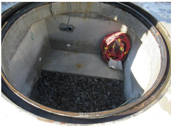
Fig.12 Inside of Manhole(10 month later)
